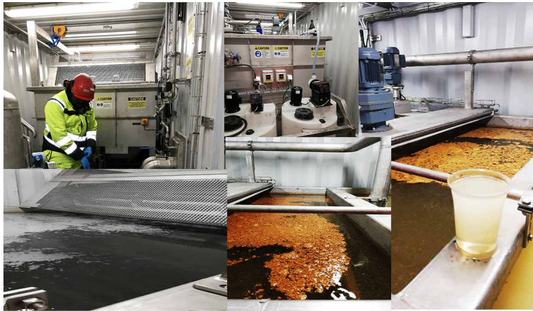
Figure 14. Validation at Kevitsa with pilot DAF test container (35000L/h). The orange and black sludge floating on the water surface comprises the impurities removed from the water.
